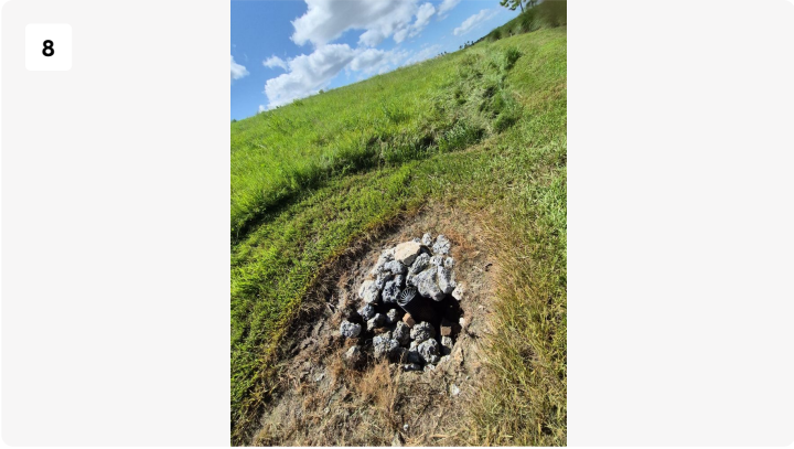
Project: 5220 - The Heights Contract Maintenance Date: Aug 18, 2026, 11:12 AM Creator: Rony Romero
