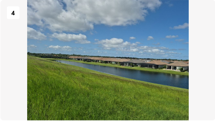
Project: 5220 - The Heights Contract Maintenance Date: Aug 18, 2026, 11:04 AM Creator: Rony Romero
