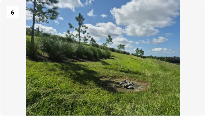
Project: 5220 - The Heights Contract Maintenance Date: Aug 18, 2026, 11:08 AM Creator: Rony Romero
