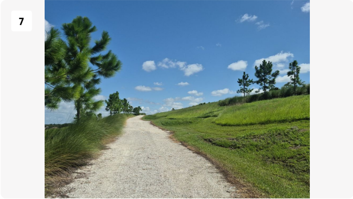
Project: 5220 - The Heights Contract Maintenance Date: Aug 18, 2026, 11:10 AM Creator: Rony Romero
