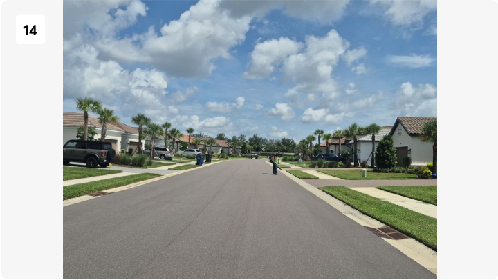
Project: 5220 - The Heights Contract Maintenance Date: Aug 4, 2026, 11:37 AM Creator: Rony Romero
