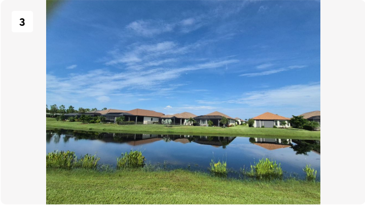
Project: 5220 - The Heights Contract Maintenance Date: Aug 4, 2026, 10:36 AM Creator: Rony Romero
