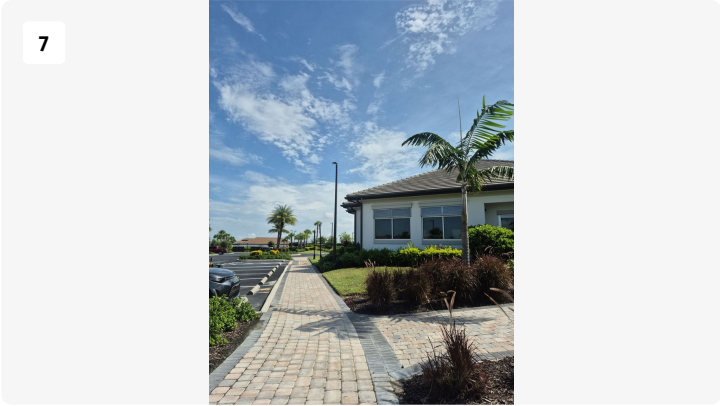
Project: 5220 - The Heights Contract Maintenance Date: Aug 4, 2026, 11:01 AM Creator: Rony Romero
