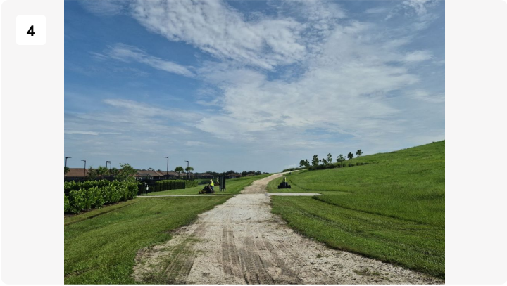
Project: 5220 - The Heights Contract Maintenance Date: Aug 4, 2026, 10:37 AM Creator: Rony Romero
