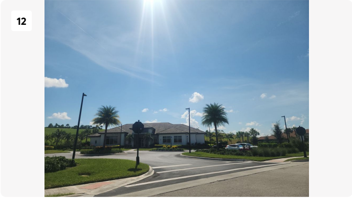
Project: 5220 - The Heights Contract Maintenance Date: Sep 15, 2026, 11:33 AM Creator: Ruben Torres-Soto
