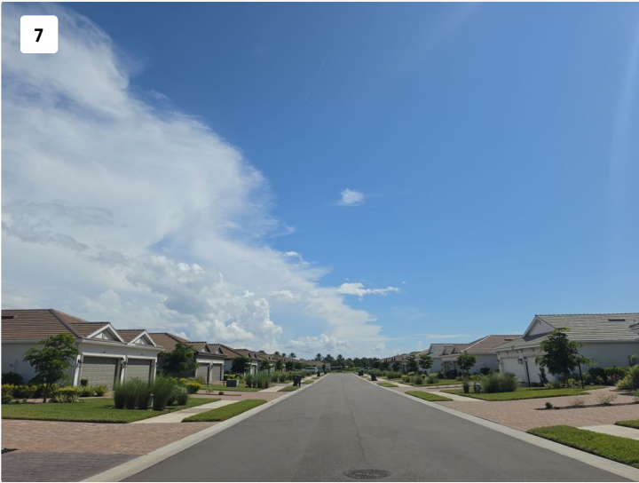
Project: 5220 - The Heights Contract Maintenance Date: Sep 22, 2026, 3:30 PM Creator: Ruben Torres-Soto
